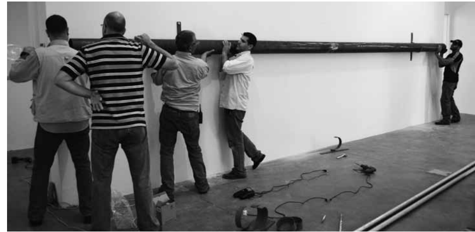
AUB Physical Plant workers installing the work of Gregory Sholette
